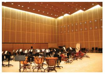
Figure 2.25: Wood-based panels used as wall linings at Copenhagen Opera House Photo: Coillte Panel Products
