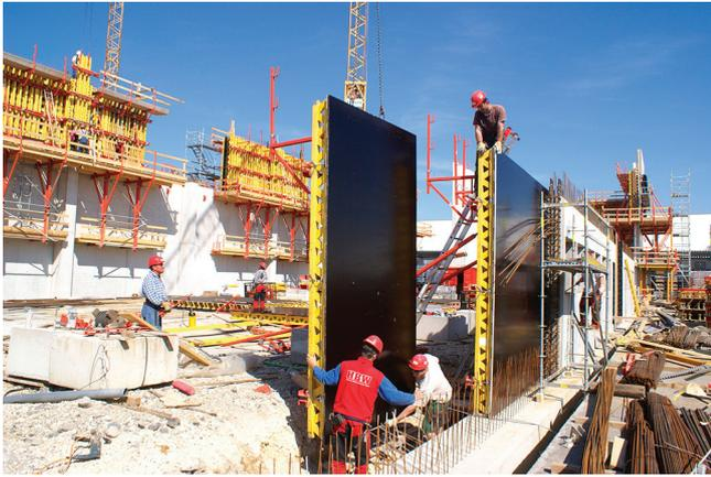
**Figure 2.19: Wood-based panels used in formwork**
