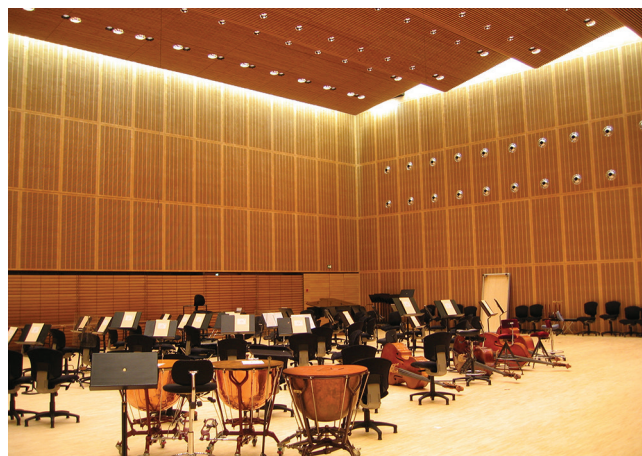
Figure 2.25: Wood-based panels used as wall linings at Copenhagen Opera House
