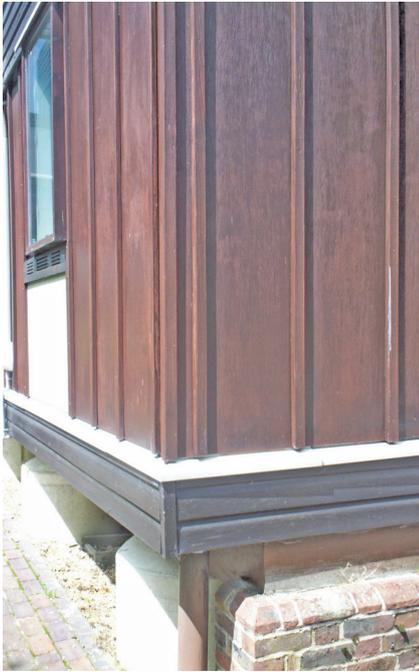
**Figure 2.20: Wood-based panels used in cladding, fascias and soffits**
