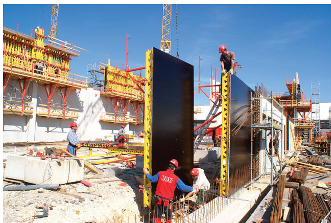
Figure 2.19: Wood-based panels used in formwork Photo: UPM-Kymmene Wood Oy
