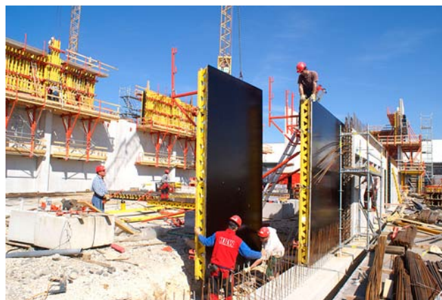
Figure 2.20: Wood-based panels used in formwork Photo: UPM-Kymmene Wood Oy
